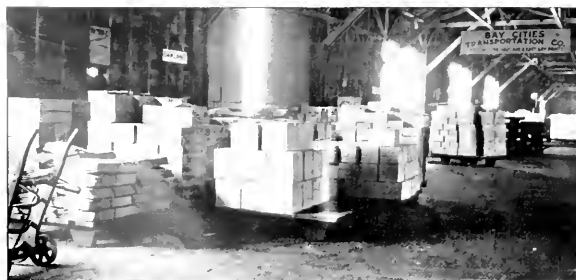
View on the dock, Bay Cities Transportation Company, showing freight stowed on platforms ready for movement.
